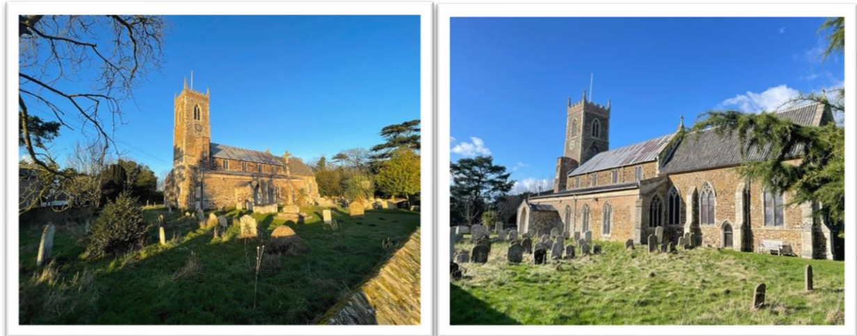
Figure 15-Pictures of the St Peter and St Paul's Church
